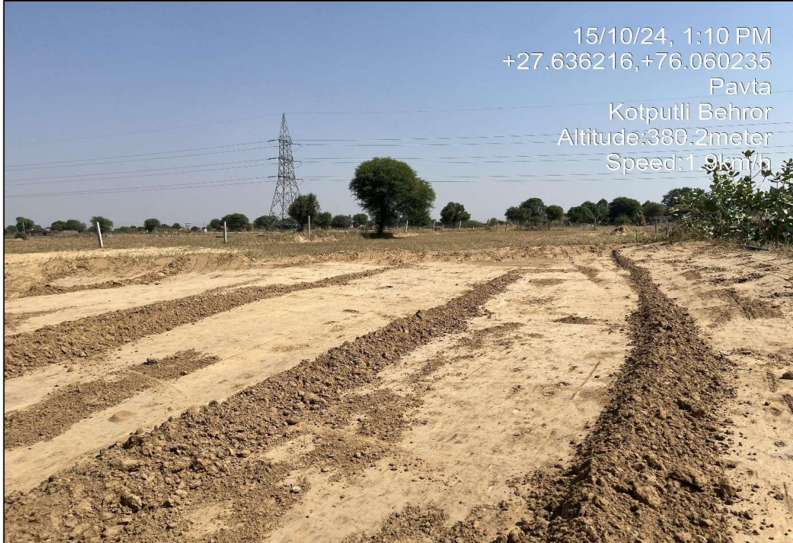
Fig 01: Khasra No. 1935, levelling work being done.
